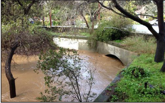
Upstream face of Pope/Chaucer Street with water surface approximately two feet below the soffit
